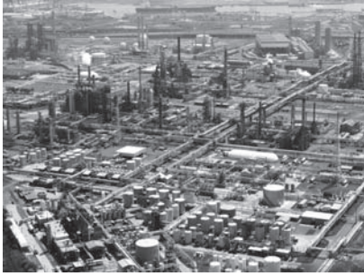
Current Bayway Oil Refinery -- Bayway, NJ
